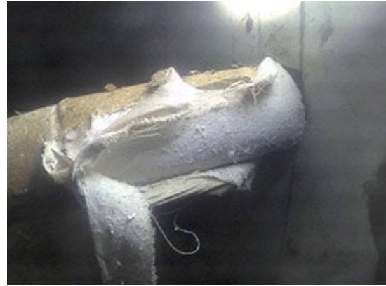
Image 8: Asbestos pipe insulation
