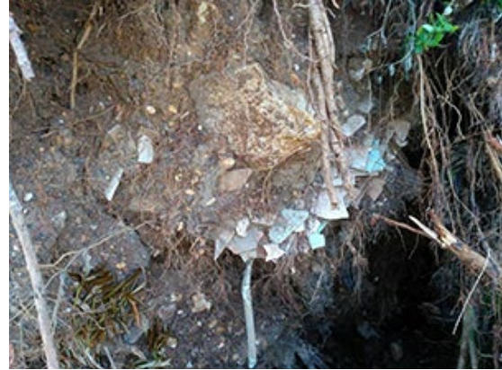
Image 16: Legacy asbestos in tree roots
