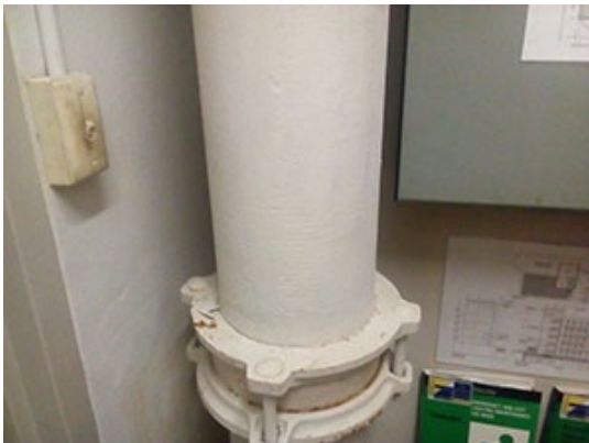
Image 35: Asbestos piping
