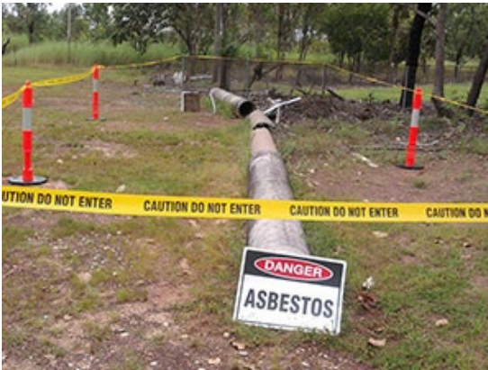
Image 9: Asbestos pipes
