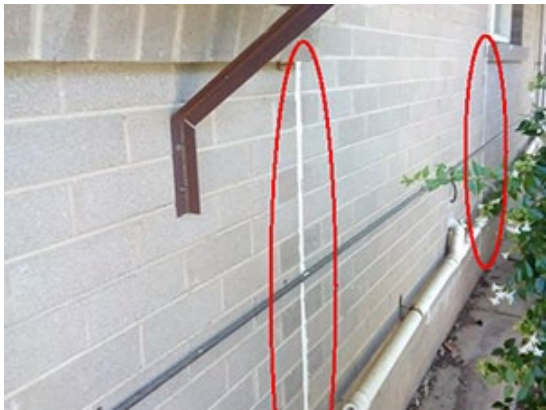
Image 25: Asbestos expansion joint sealants
