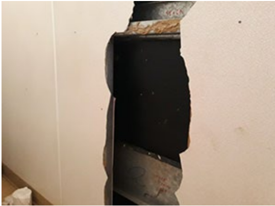
Image 23: Black sound deadening paint behind urinal
