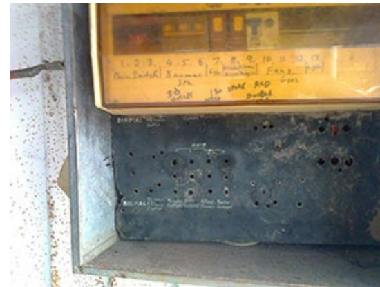
Image 14: Asbestos backing board
