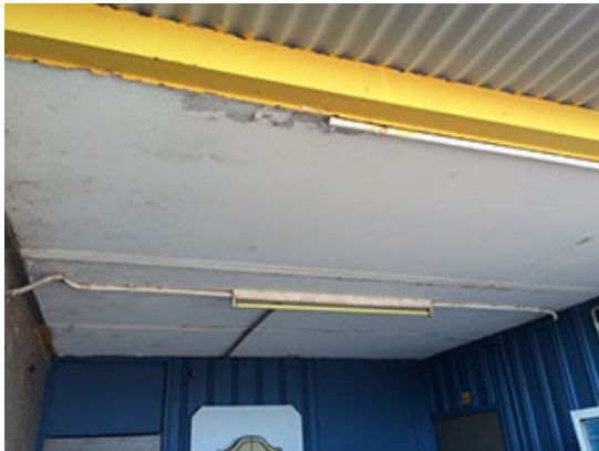
Image 41: Asbestos refrigeration panel ceiling and walls
