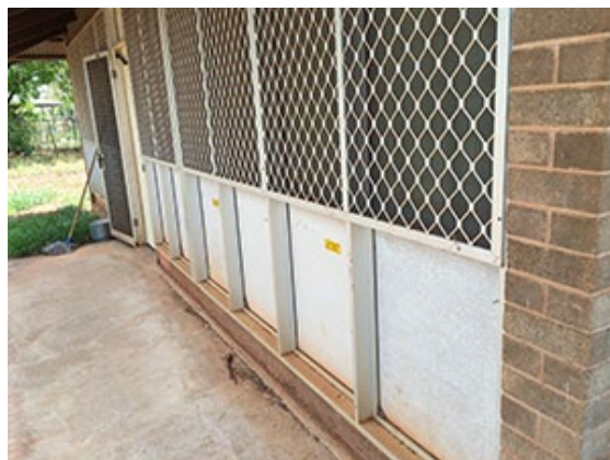
Image 45: Window infill panels
