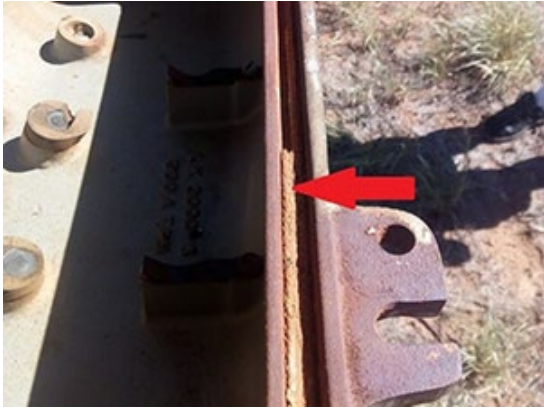
Image 1: Asbestos packer
