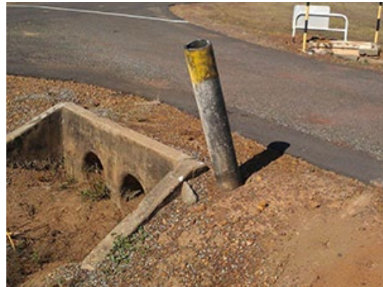
Image 2: Asbestos bollard
