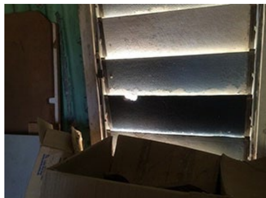
Image 6: Asbestos louvers
