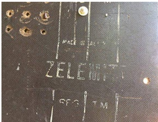
Image 13: Asbestos zelemite in meter box
