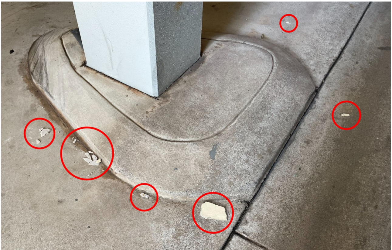
Image: Small pieces (fragments) of ACM at the entrance of a building's carpark.
