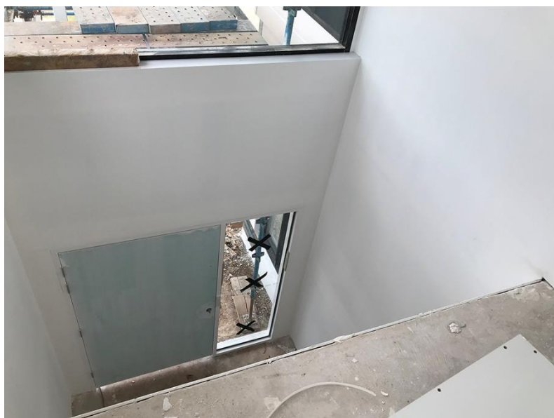
Image 1: Unguarded voids are a serious risk to workers health and safety.
