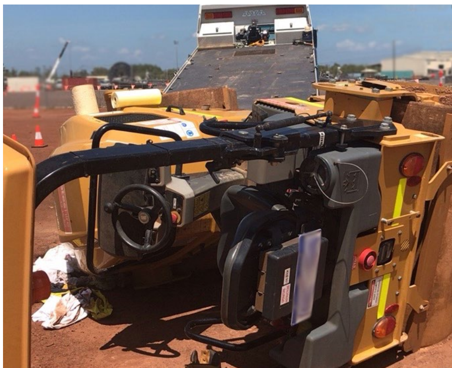
Image: The 2.7 tonne compactor in situ after toppling.
