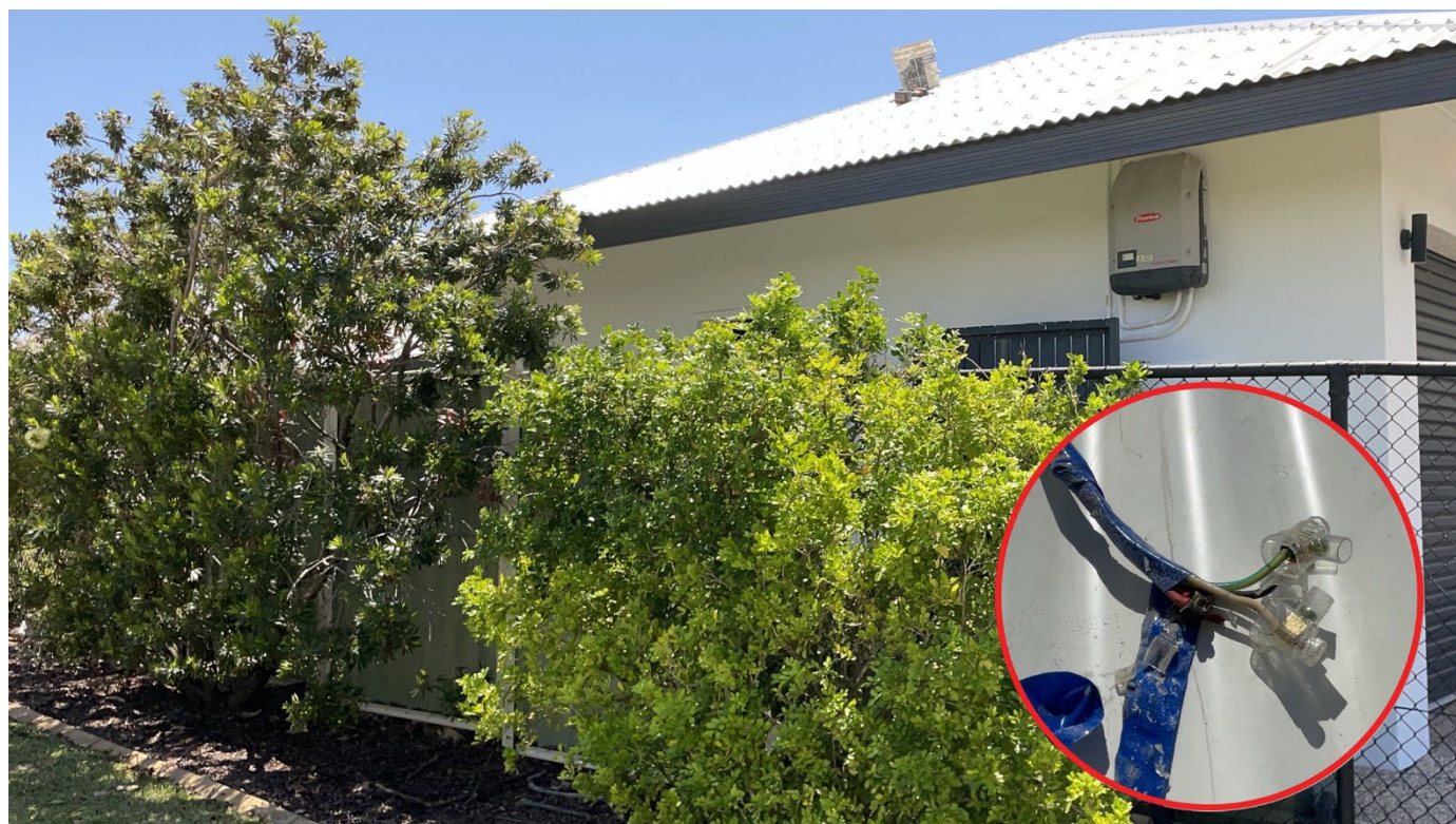
Image: The apprentice fell from the roof, onto the fence and landed in the neighbouring yard after an electric shock. (Insert) A connector used to insulate the wiring was damaged, exposing live parts.
