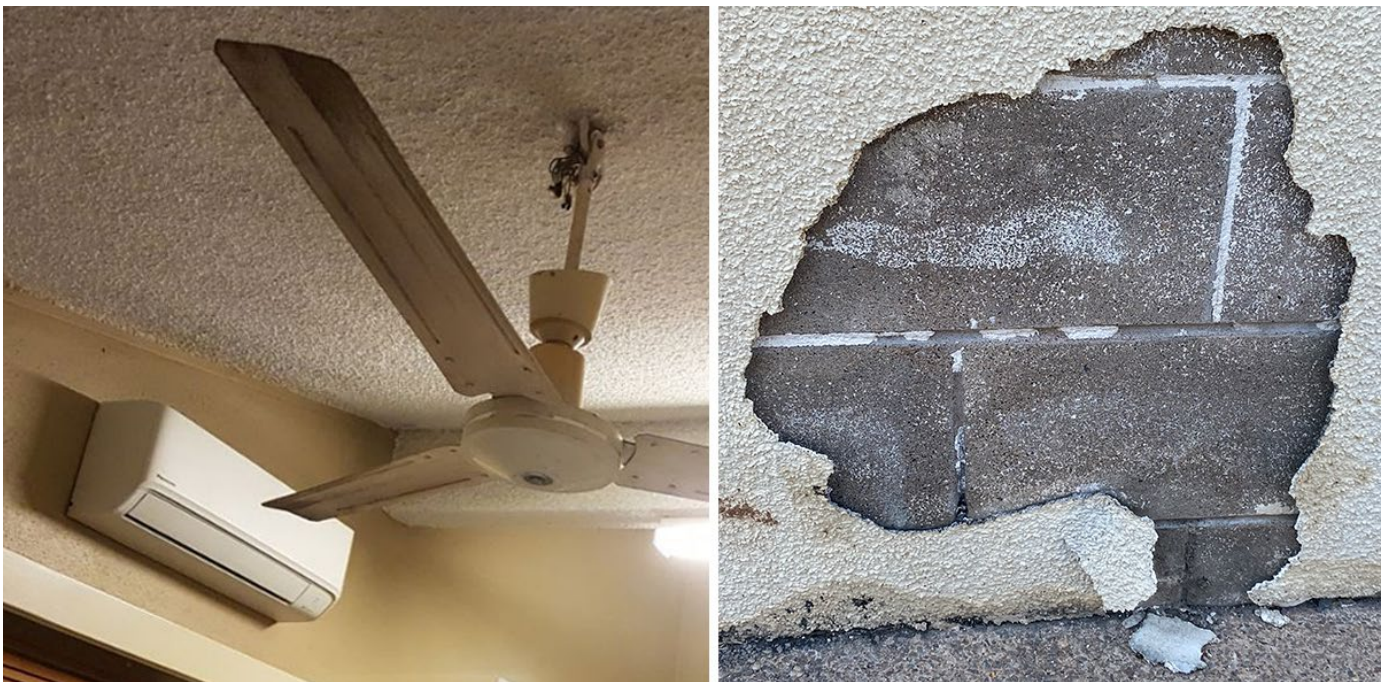
Image: The asbestos containing vermiculite (left). The asbestos containing external render (right).
