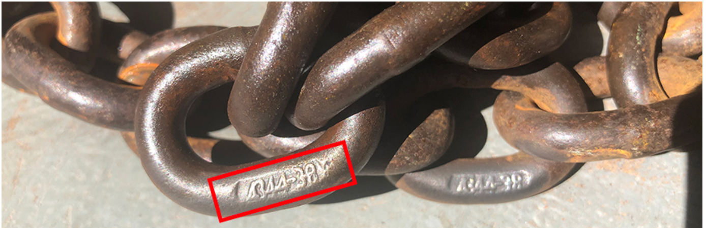
Image 1: The 4344-38 identification marking on this chain means it complies with Australian Standard 4344 and has a 3.8 tonne capacity.
