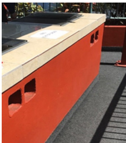
Image 1: Ventilation points at the top still of the compartment still allowed gas to accumulate at the bottom.
