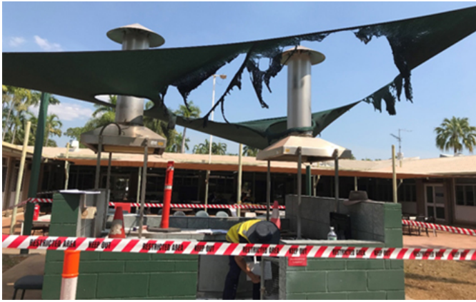
Image 2: The wall enclosing the barbecue facility blocked flow through ventilation allowing gas to accumulate.
